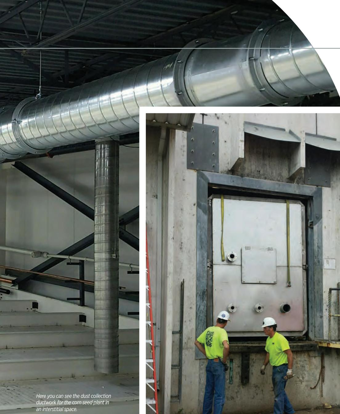
Here you can see the dust collection ductwork for the corn seed plant in an interstitial space.
