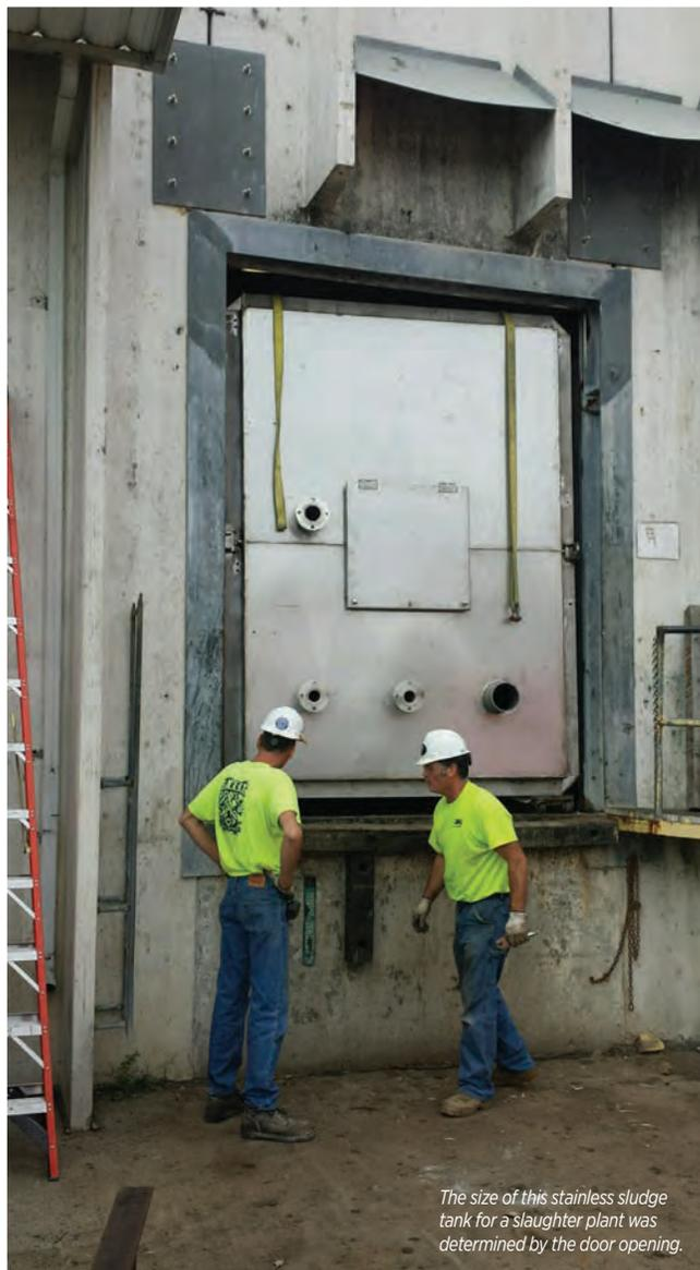
The size of this stainless sludge tank for a slaughter plant was determined by the door opening.
