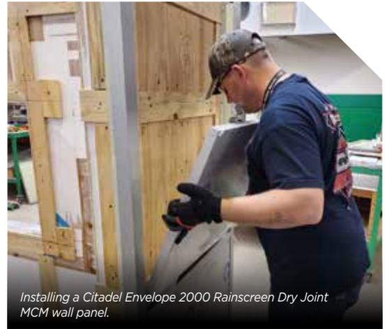
Installing a Citadel Envelope 2000 Rainscreen Dry Joint MCM wall panel.
