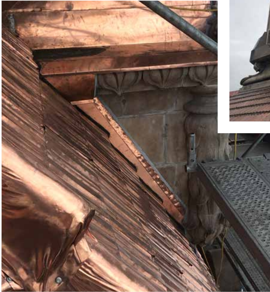
LEFT and FAR LEFT: The Sun Tower is a Vancouver landmark that's been around since 1912. Originally topped with terracotta tiles that were painted green, everyone thought they were made of copper. As the terracotta tiles deteriorated, copper was the most cost-effective, long-lasting replacement.
