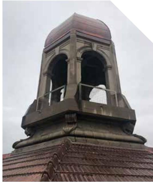
LEFT and FAR LEFT: The Sun Tower is a Vancouver landmark that's been around since 1912. Originally topped with terracotta tiles that were painted green, everyone thought they were made of copper. As the terracotta tiles deteriorated, copper was the most cost-effective, long-lasting replacement.
