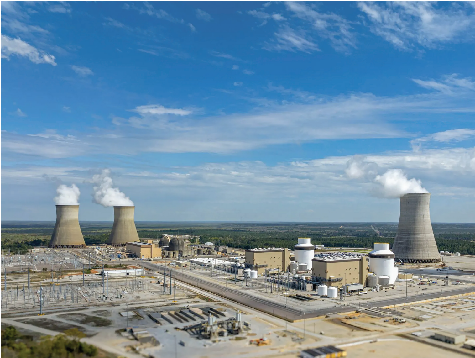
Plant Vogtle, located in Waynesboro, Georgia, is the largest generator of clean power in the United States. Photo: Georgia Power
