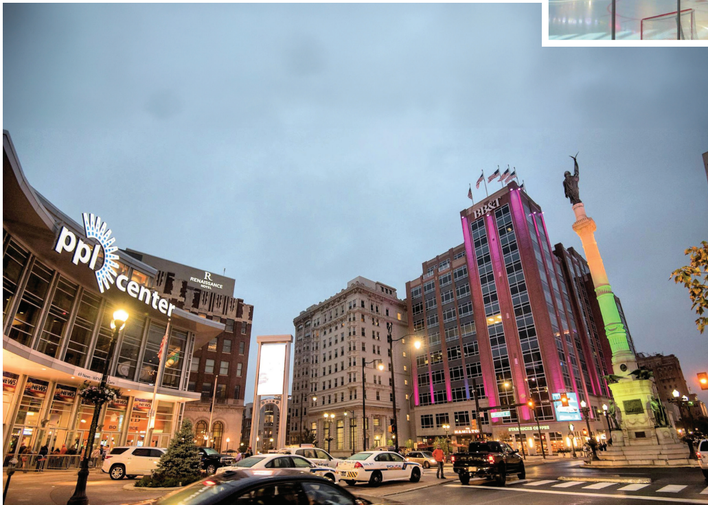
The PPL Plaza includes a LEED Gold, 8-story office building, Renaissance Allentown Hotel, and an array of shops and restaurants.
