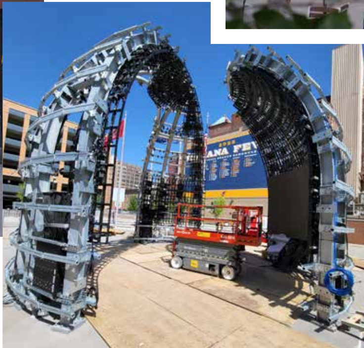
Physical assembly of the structures was challenging. The arch had 450 pieces, and the sphere had more than 350 panels.
