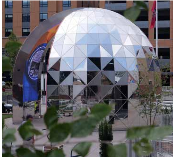
Physical assembly of the structures was challenging. The arch had 450 pieces, and the sphere had more than 350 panels.
