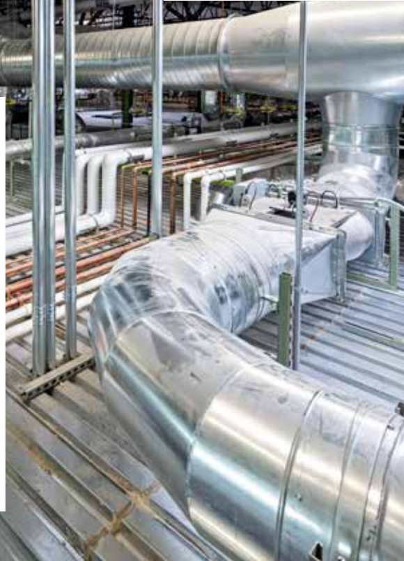
Apollo Mechanical installs 190,000 pounds of new galvanized and stainless steel at the North Valley Complex in Wilsonville Oregon, in addition to updating the HVAC.
