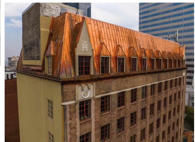
The nine-story Studio Building in Portland, Oregon, was built in 1926. Harder Mechanical replaced the aging roof with 20-ounce copper panels.
