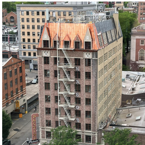
Harder Mechanical was able to update a nearly century old building in Portland, Oregon, while maintaining its historical significance.
