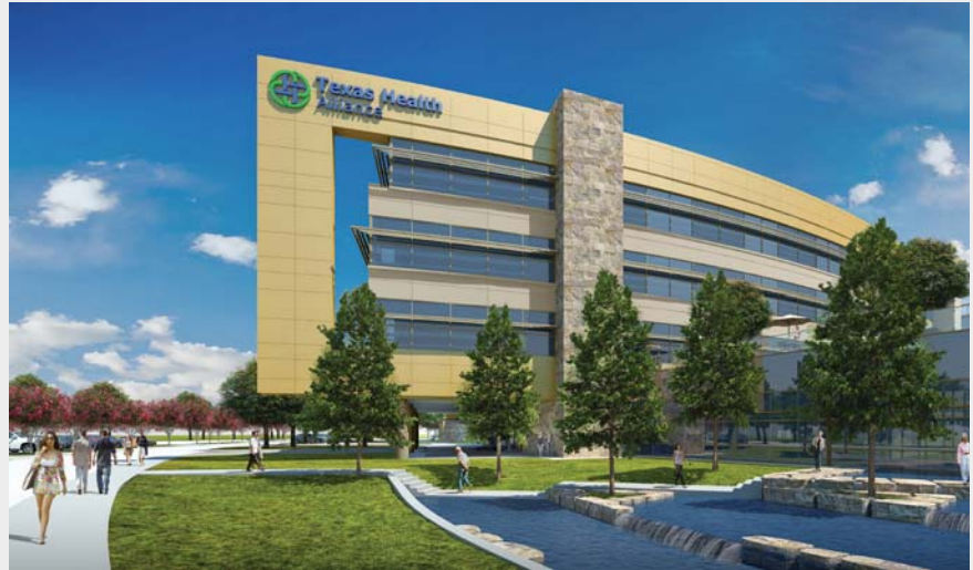
The hospital will feature multi-trade prefabricated racks in the corridors, an approach that is still new in the U.S.
